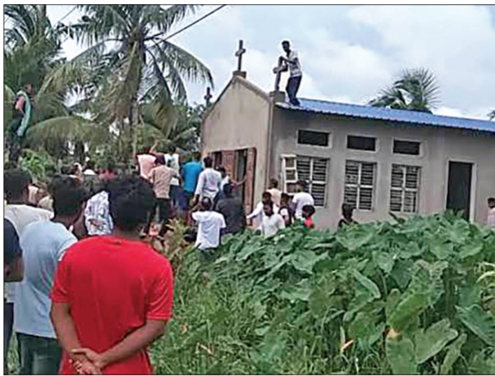
The mob attack on this newly built church in Subhasgram (South 24 Parganas) on 5 July was among the first incidents that set off the trend
